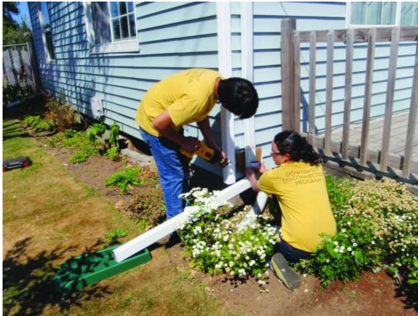
Roof top disconnect
